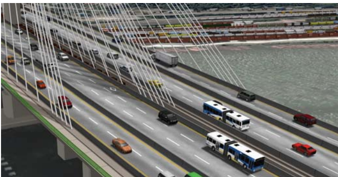
Artist's rendering of the new Port Mann Bridge showing transit/HOV lanes and separation of through traffic from local traffic.
