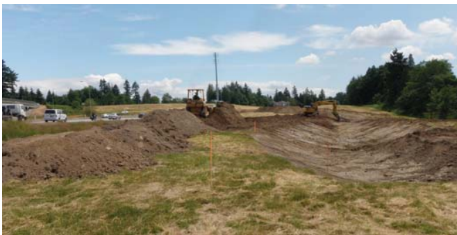
Surrey - Environmental enhancement work at 160th Street.
