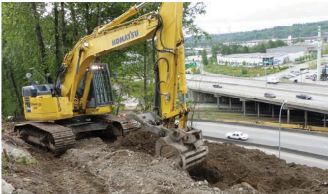
Coquitlam - Lougheed Highway cut near the Cape Horn Interchange.
